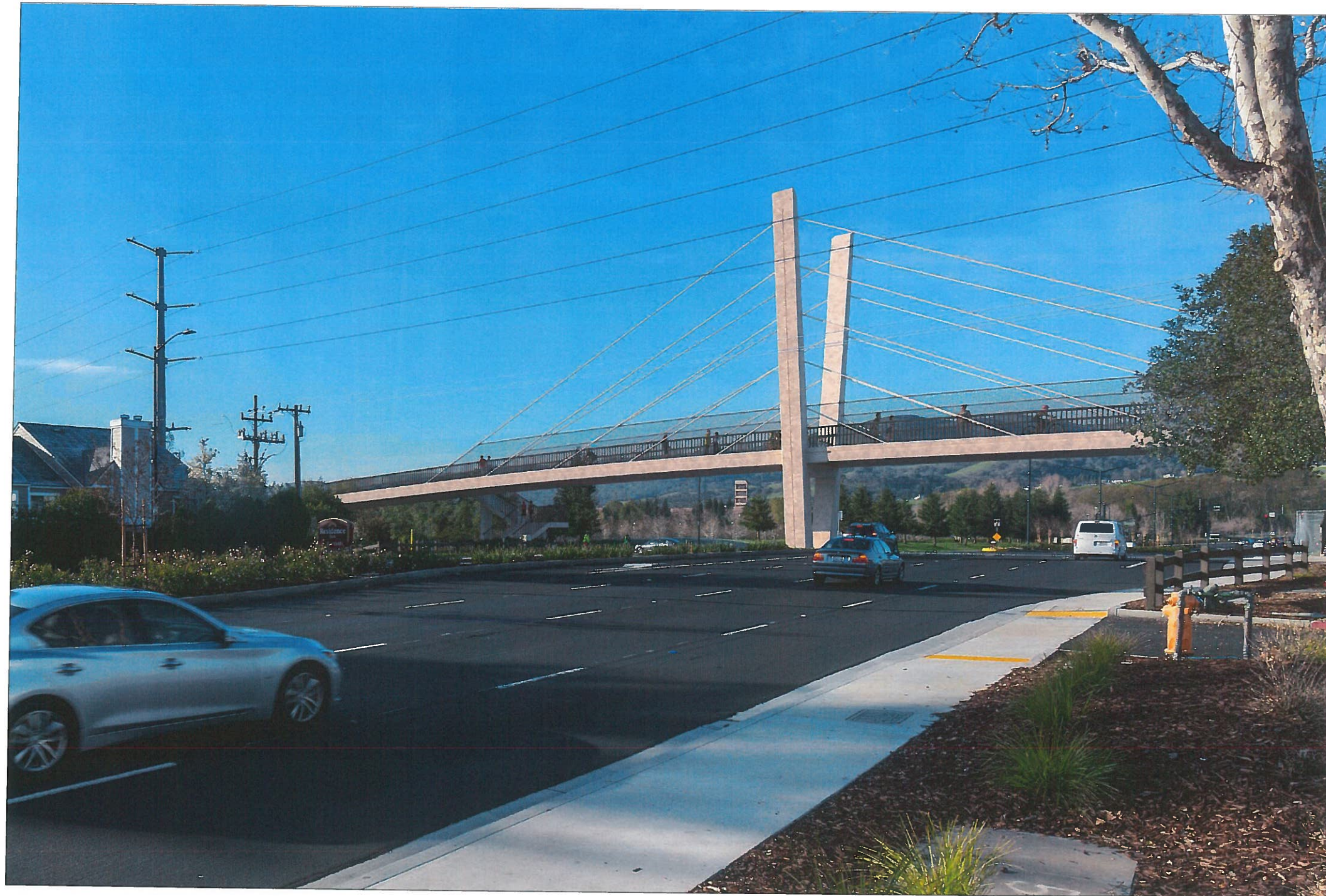
PLATE P02 OPTION 1 - CABLE STAY, PYLON ON BOLLINGER CANYON ROAD MEDIAN
