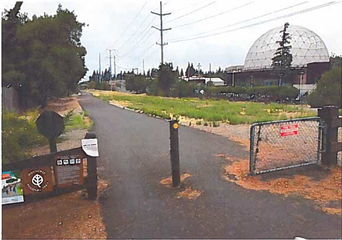
Photo 3: Existing Iron Horse Trail, North of the Crow Canyon Road Crossing
