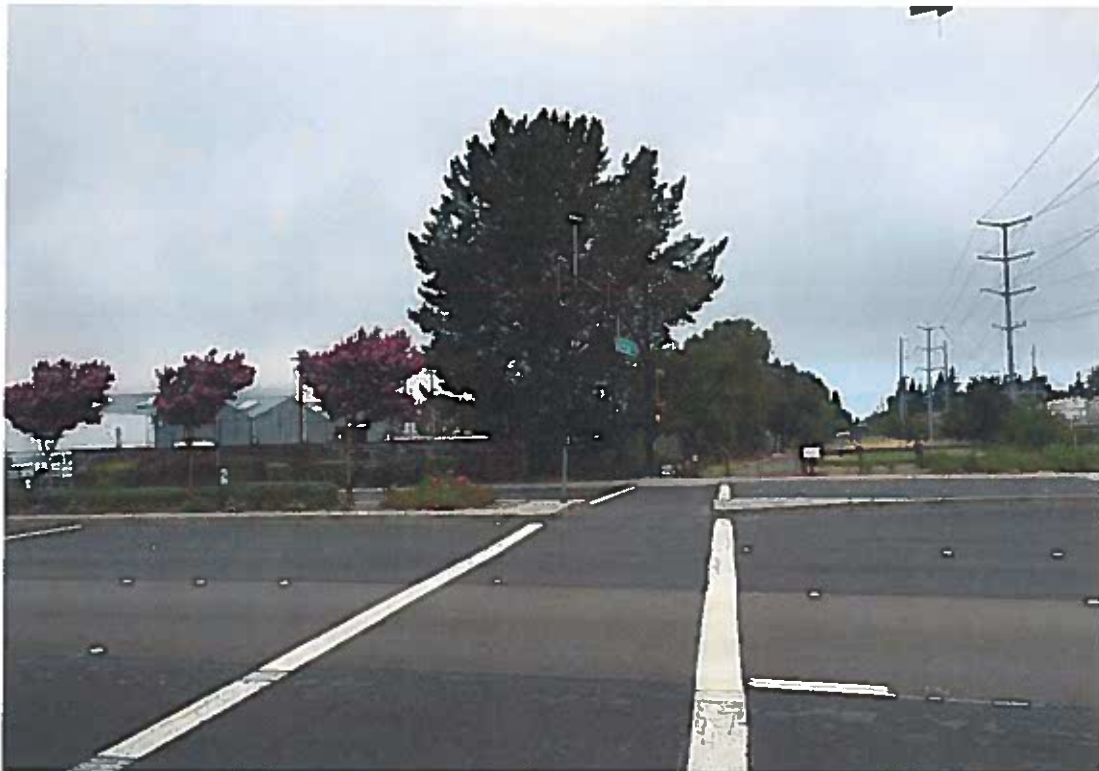
Photo 2: Existing Iron Horse Trail Crossing at Crow Canyon Road, Looking North
