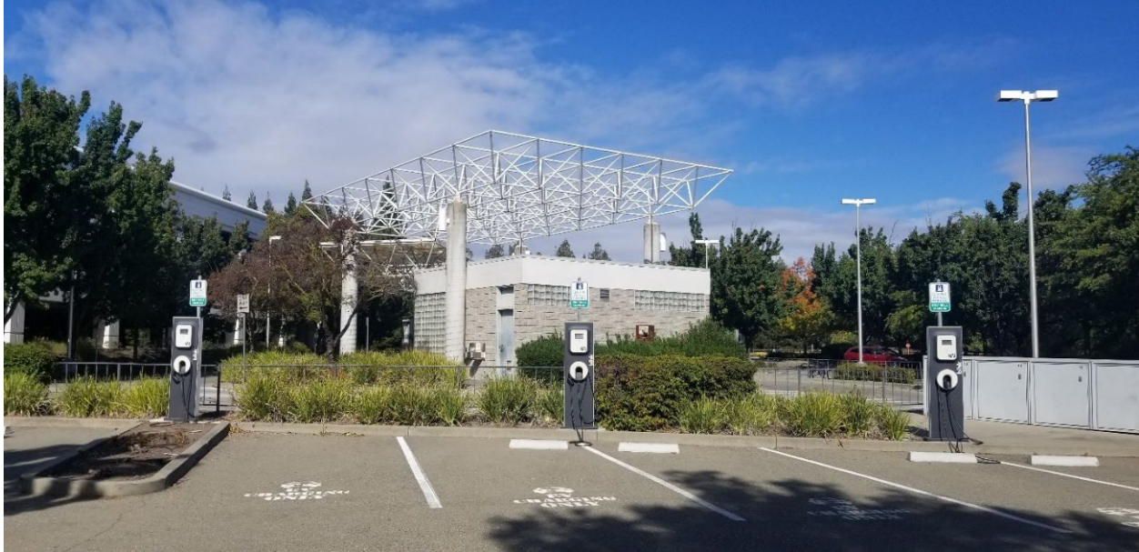
Figure 32. San Ramon Transit Center EV Charging Stations
