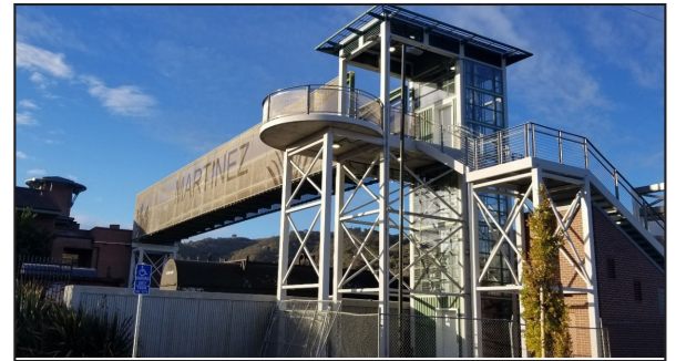
Figure ES-7. Pedestrian Bridge at Martinez Amtrak Station
