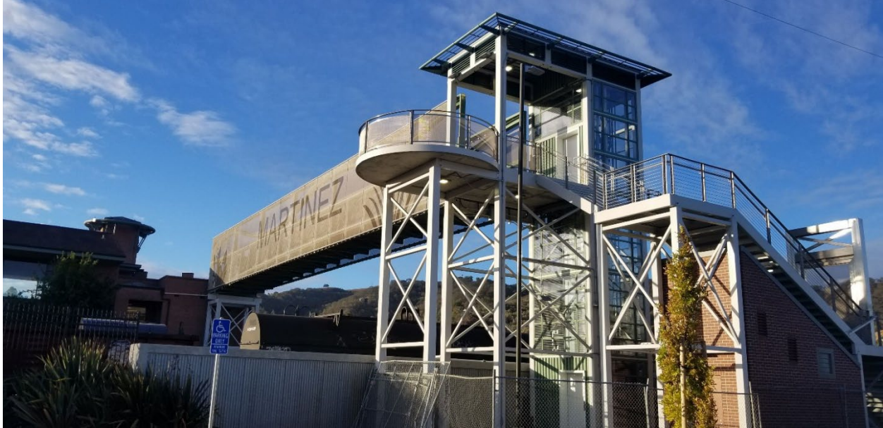
Figure 18. Pedestrian Bridge at Martinez Amtrak Station
