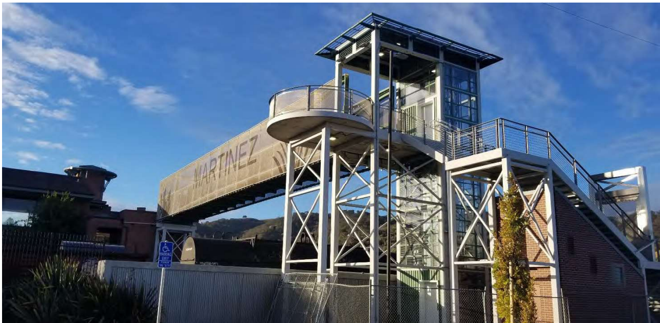
Figure 4. Pedestrian Bridge at Martinez Station
