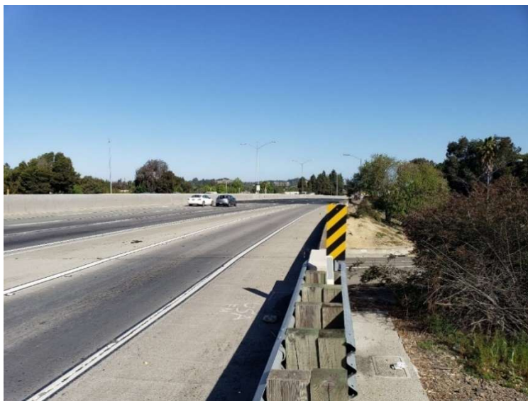
Figure 4-7 The Existing Burnett Avenue On-Ramp Merge and Concord Avenue Overpass
