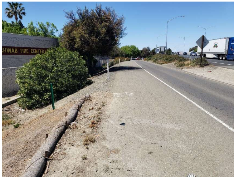
Figure 4-9 Concord Avenue / Chilpancingo Parkway On-Ramp (looking north)
