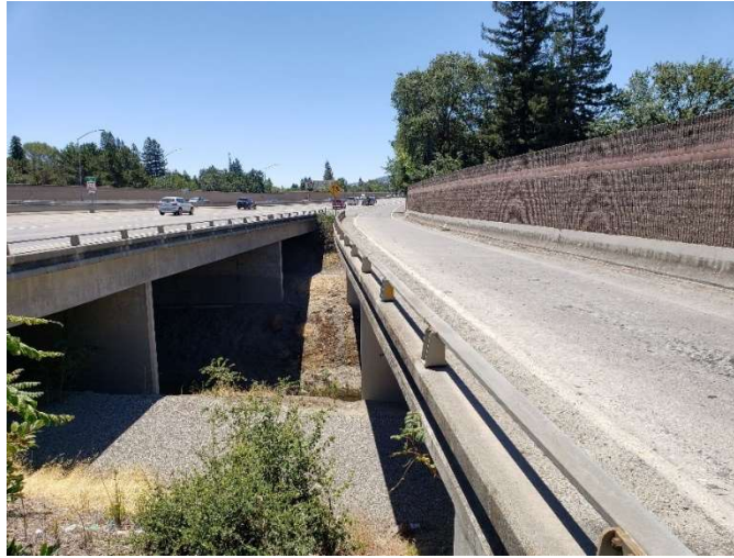
Figure 4-17 Diablo Road On-Ramp Crossing San Ramon Creek
