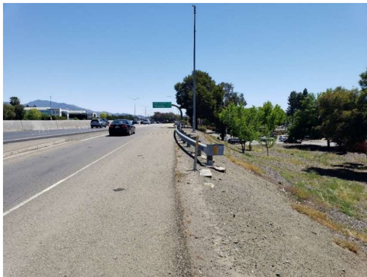
Figure 4-8 Contra Costa Boulevard On-Ramp Merge with I-680 Southbound
