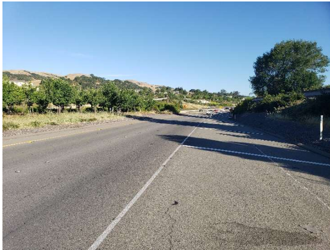
Figure 4-5 Additional Paved Area on Alcosta Boulevard On-Ramp
