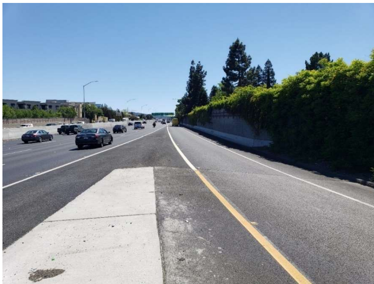
Figure 4-12 Existing San Luis Road / North Main Street Sound Wall and Merge with I-680 SB
