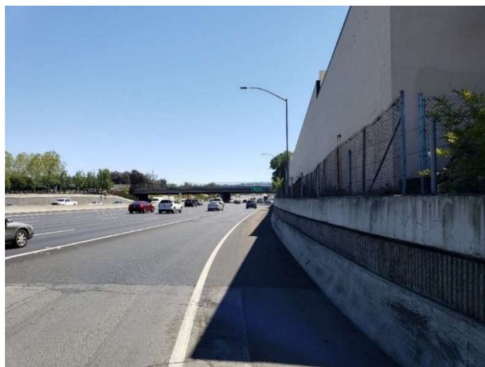
Figure 4-11 Commercial Building and Retaining Wall at the North Main Street / Sunnyvale Avenue On-Ramp
