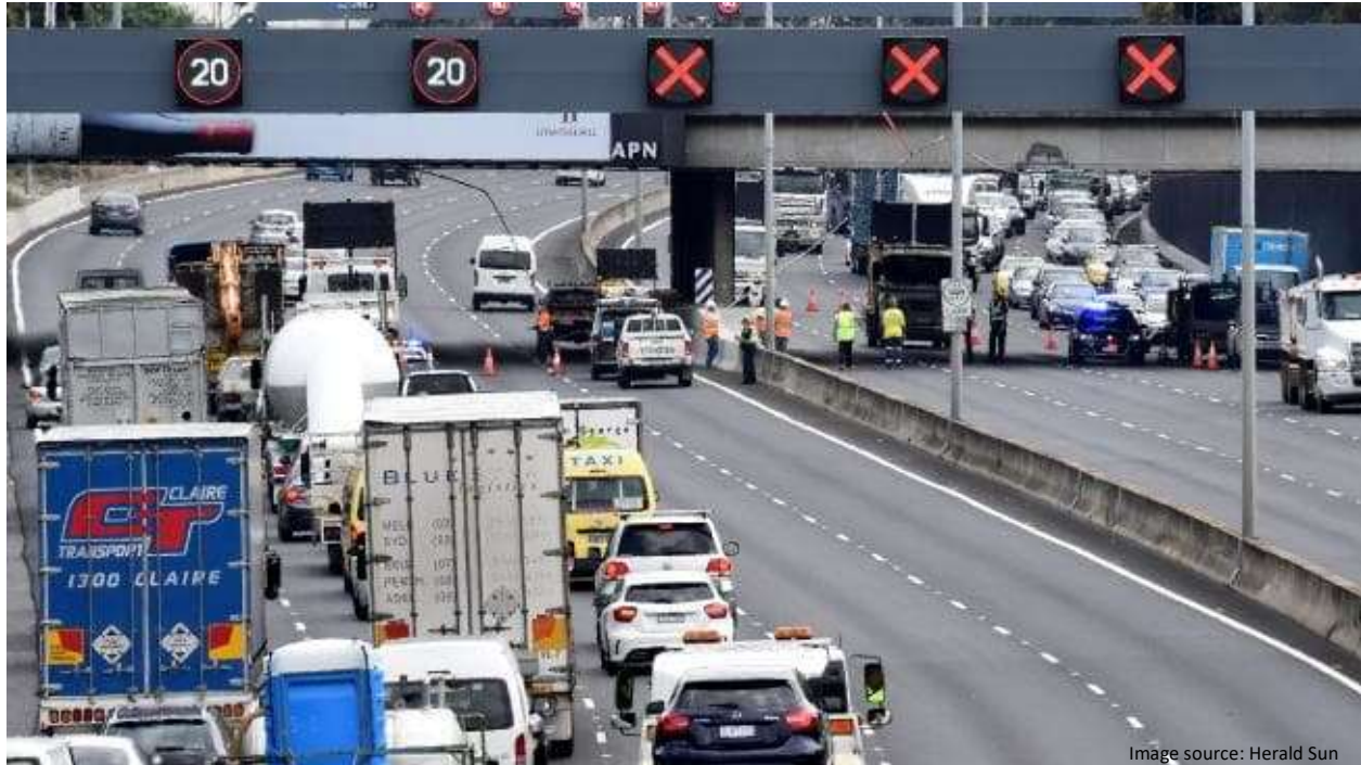
Figure 2-9 Lane Use Management System on M2 Tullamarine Freeway, Melbourne, Australia
