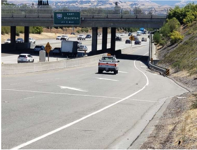
Figure 4-18 San Ramon Valley Boulevard On-Ramp Lane Merge and Alcosta Boulevard Undercrossing
