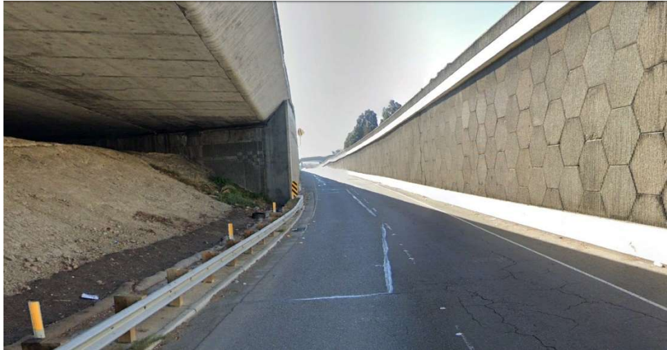
Figure 4-13 Existing I-680 Southbound On-Ramp at Hillside Avenue / Ygnacio Valley Road
