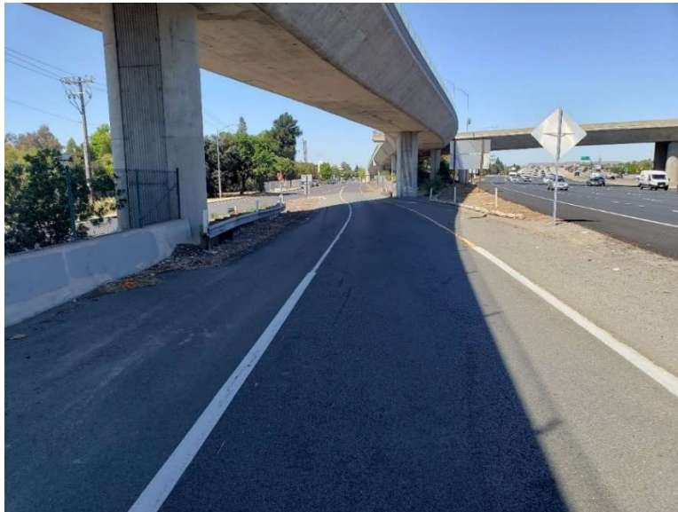
Figure 4-10 Boyd Road / Contra Costa Boulevard Access Ramp to I-680 Southbound (looking north)
