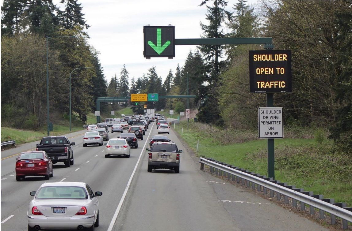
Figure 7-9 Example Part-Time Shoulder Lane Use Management System, I-405 near Seattle, Washington
